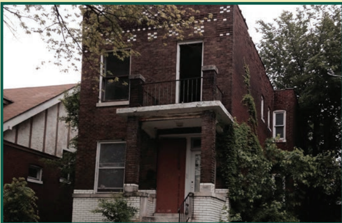
TGNCDC purchased the long-vacant and failing building at 3719 Bamberger Ave. from an out-of-town “investor,” rebuilt the facade and added a new thermoplastic polyolefin roof. It was then sold to Jeff Sutton from Bloomsdale Development, who finished the renovation into two 2-bedroom apartments.
